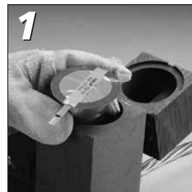
1 Insert CADWELD PLUS package into mould
