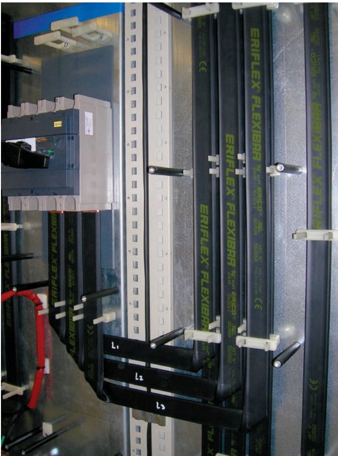
Application pictures: Flexibar directly connected on various devices or rigid bars, with compact connection and from 125 A up to 4500A.
