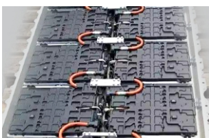
Battery charge/discharge test
