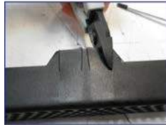
Cut holes to allow cable access
