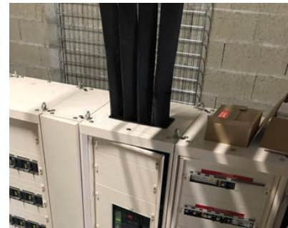
Example of global cut out on magnetic plate (steel)
