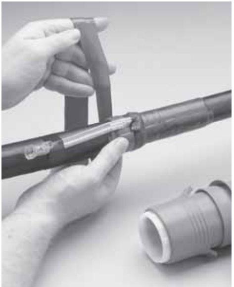
Photo 8: Apply the sealant tape below the stress control patch.
