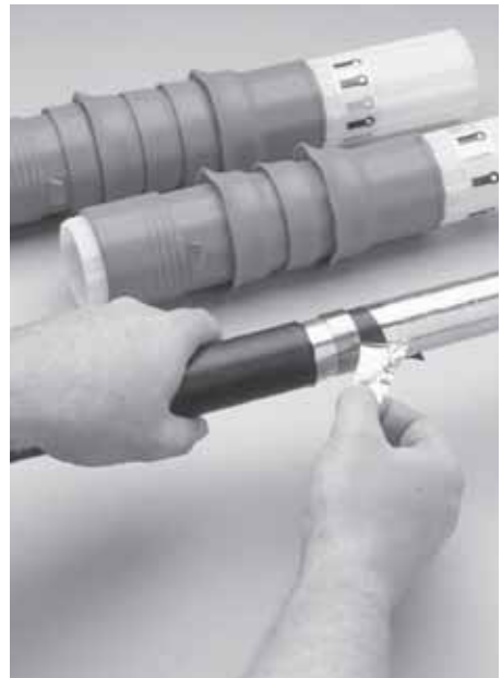
Photo 4: Using the roll clip to cut and remove the copper screen.
