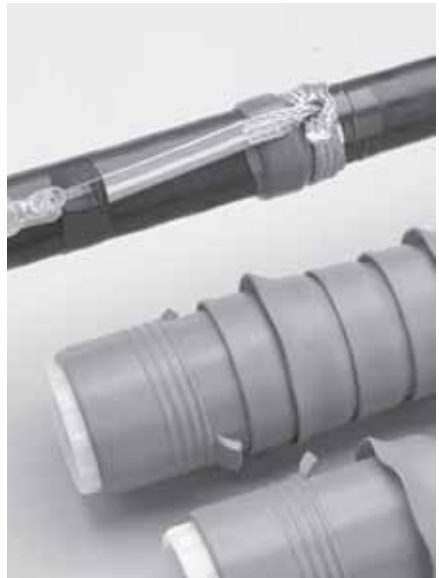
Photo 6: Bonding braid secured in place.
